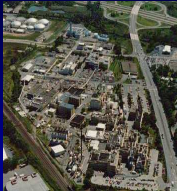
Chemical Process Plant
